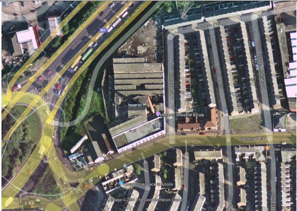
Monarch Laundry site prior to demolition
